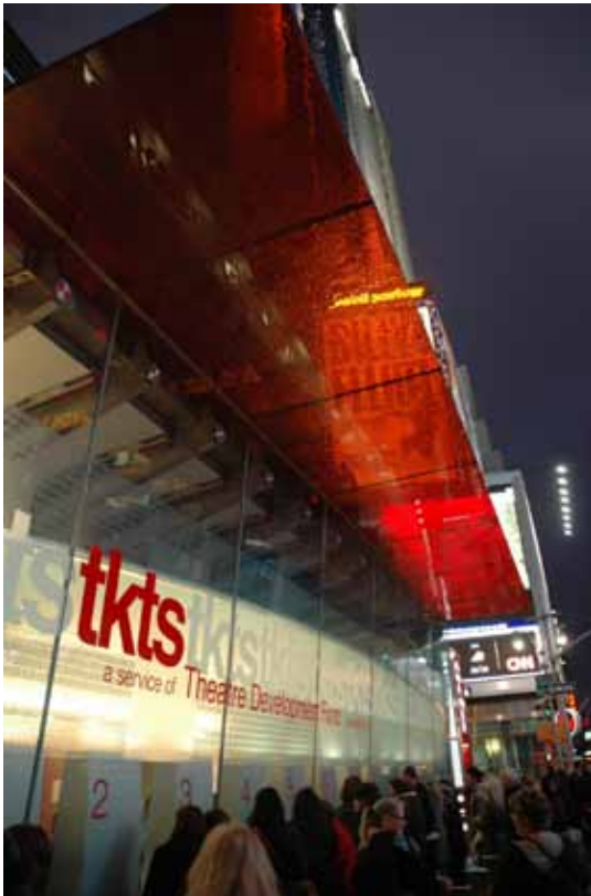
SentryGlas® ionoplast interlayers enable innovative frameless facade and canopy design, with novel glass structural support at the TKTS booth in New York City's Times Square.
