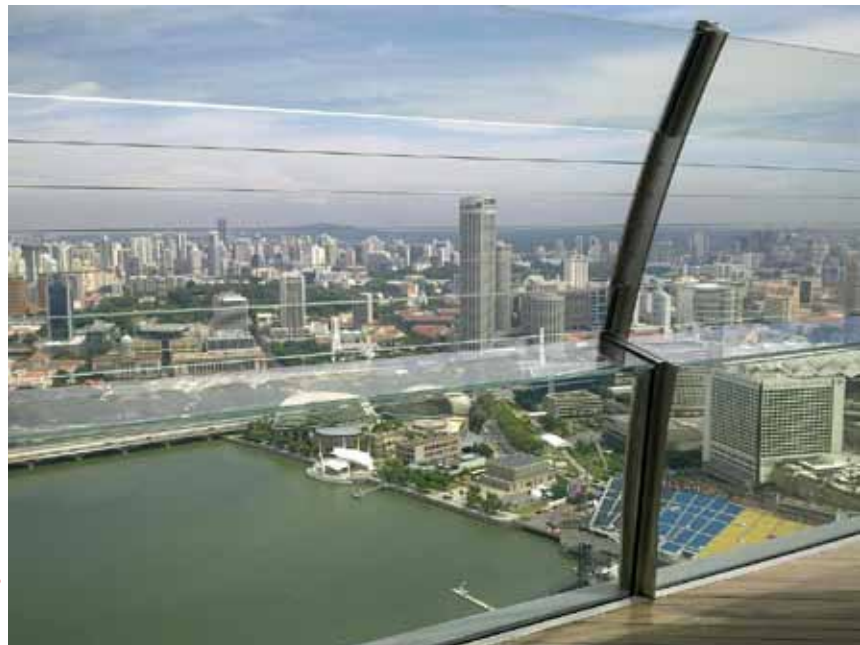
Open-edged rooftop glass railings made with DuPont™ SentryGlas® help protect people and the view at the Marina Bay Sands SkyPark in Singapore..
